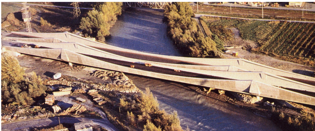
Figure 1: General view of the two Riddes bridges
