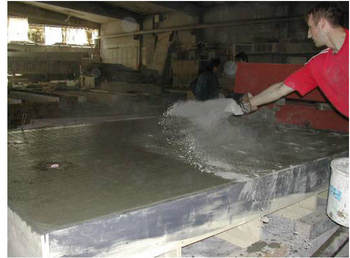
Figure 32 : Finition de la surface.
