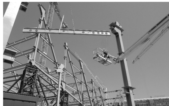
Figure 1. The structure of JTI headquarters in Geneva, with SOM, Chicago : environ 25'000 m 2 of slabs supported in only seven points, creating a 60 m long cantilever on the north-east side and a bridge like building on the west side, spanning 80 m. On the right: construction phase; in order to guarantee the geometry of the building with extremely low tolerances, the erection phases were more complex than those of any ordinary bridge structure.
