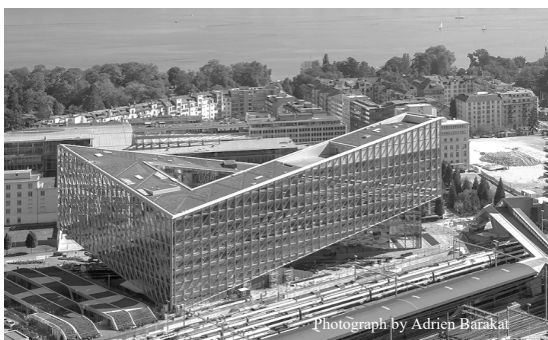
Figure 1. The structure of JTI headquarters in Geneva, with SOM, Chicago : environ 25'000 m 2 of slabs supported in only seven points, creating a 60 m long cantilever on the north-east side and a bridge like building on the west side, spanning 80 m. On the right: construction phase; in order to guarantee the geometry of the building with extremely low tolerances, the erection phases were more complex than those of any ordinary bridge structure.
