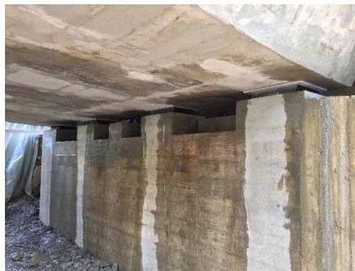
Figure 2. Refurbishing and seismic retrofitting of the CERN ISR Bridge (Synaxis SA Lausanne civil engineers).
