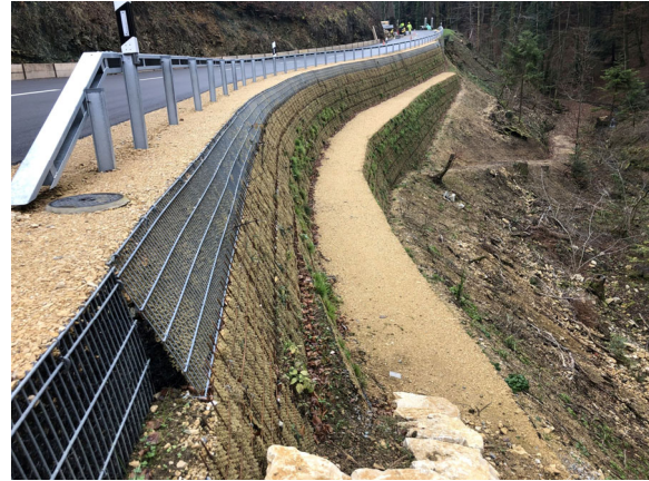
Figure 3. Left: Design sketch of reinforced soil retaining walls as an alternative to conventional RC walls (D. Tasevski, Emch+Berger AG Bern). Right: Photo of similar application of the TerraMur system (SYTEC AG).
