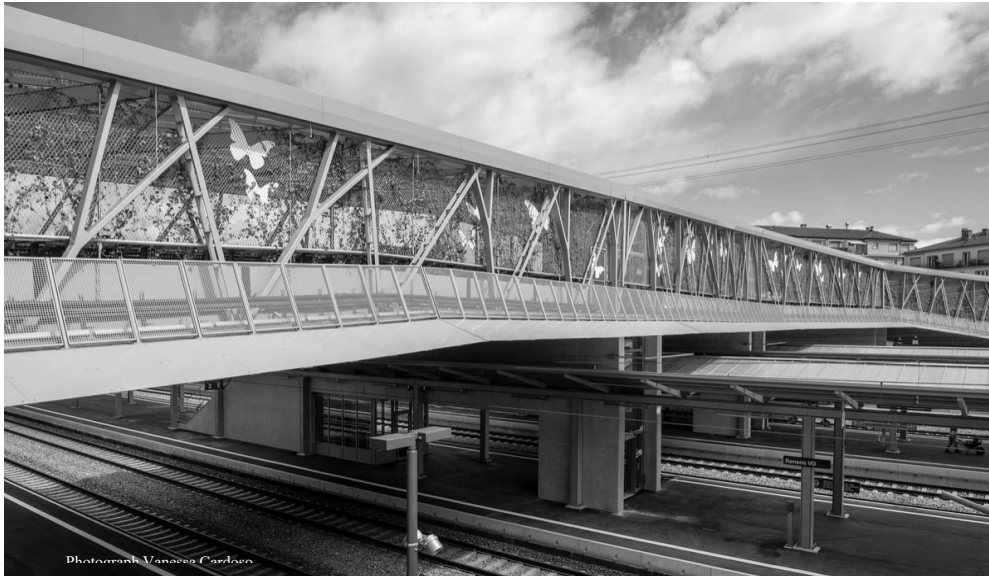
Figure 2: Passarella "Rayon vert", Renens, VD, CH, with Farra Zoumboulakis architects. It animates the passageway over the Renens SBB railway, and provides a "freshness" to the neighbourhood. The arborisation of the diagonals was a design and manufacturing challenge, as was the installation of the complete sections above the rails. The compression diagonals are bifurcated, while the tension diagonals are double plates.
