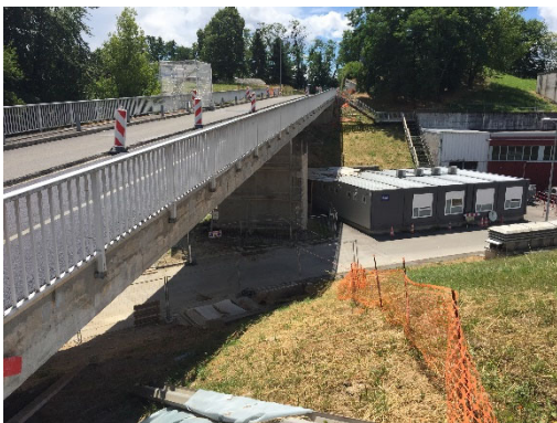
Figure 2. Refurbishing and seismic retrofitting of the CERN ISR Bridge (Synaxis SA Lausanne civil engineers).
