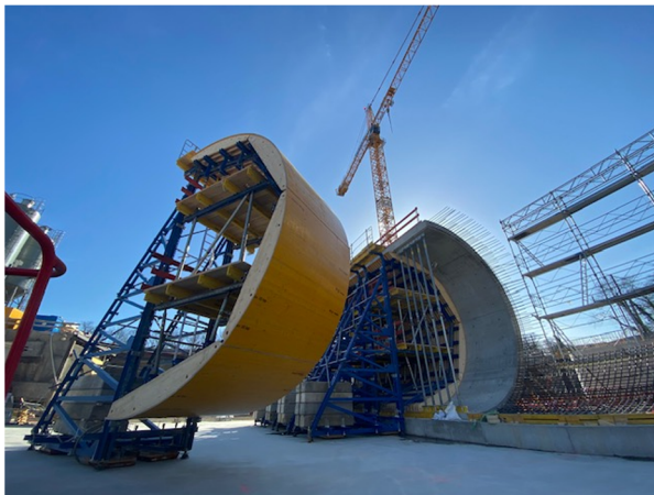
One Roof: Construction of the auditorium: formwork (on the left) finished load carrying structure (on the right)
