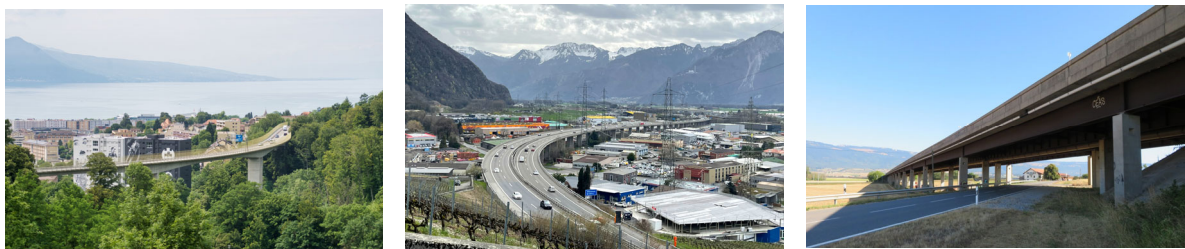
Figure 1. Extract of some bridges, which undertook a refined assessment and/or retrofitting
