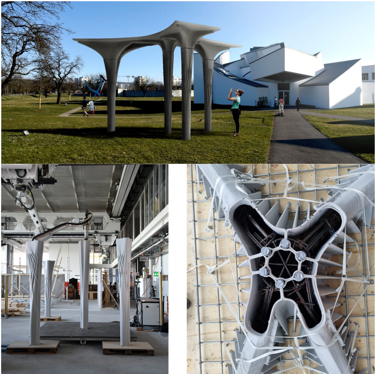
Eggshell Pavilion 3D rendering (above) printed eggshell formwork (below)
