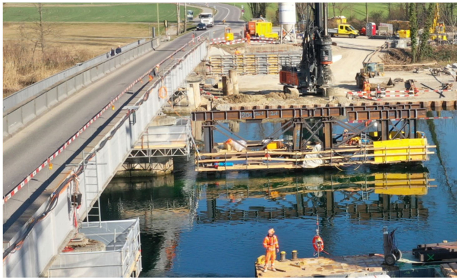
Figure 3. Picture of a temporary support before moving of the existing bridge.
