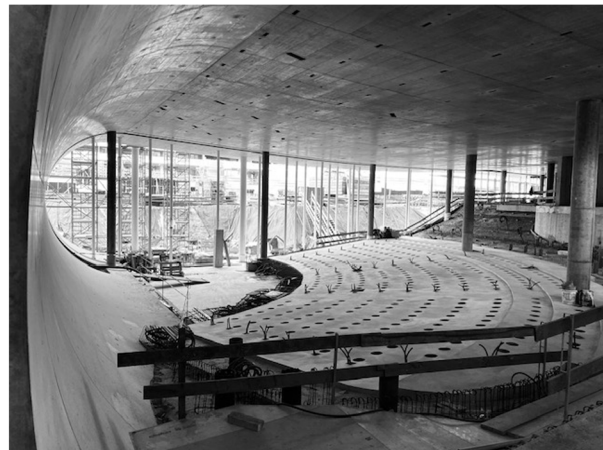
One Roof: Construction of the auditorium: formwork (on the left) finished load carrying structure (on the right)
