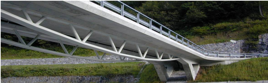
Figure 5: Tensile members for underspanned structures, possible replacement of a metallic tie by a UHPC pre-stressed member [5]
