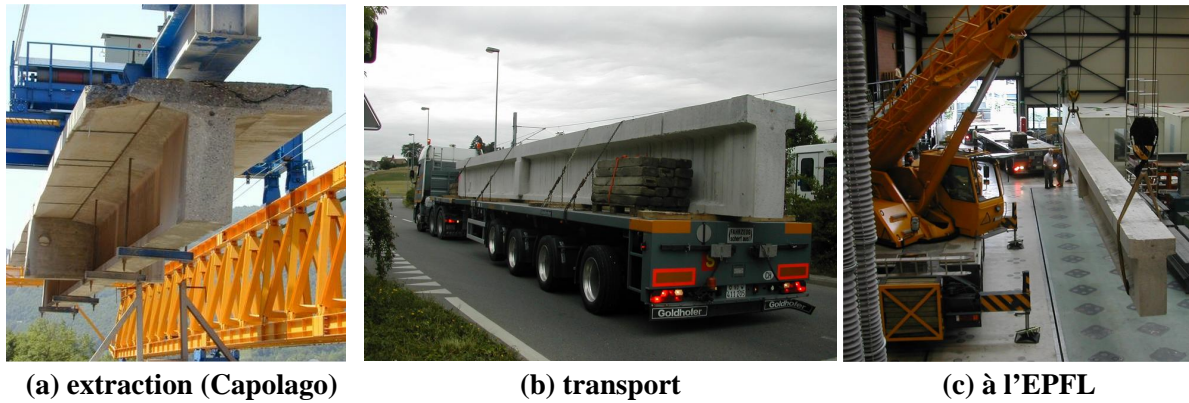
Figure 2.9: Manipulation des poutres
