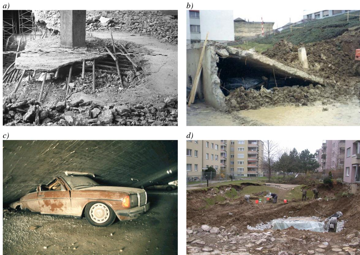
Figure 1.1: Cases of structural collapse due to punching shear failure
