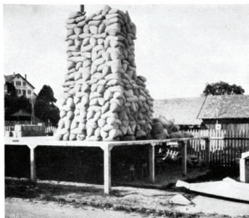
Figure 2.9: Full scale test of slab over columns, 1908, R. Maillart (Maillart 1926)
