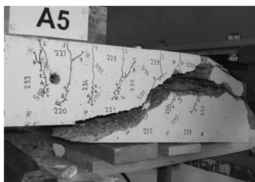
a) Shear failure of test A5V1
