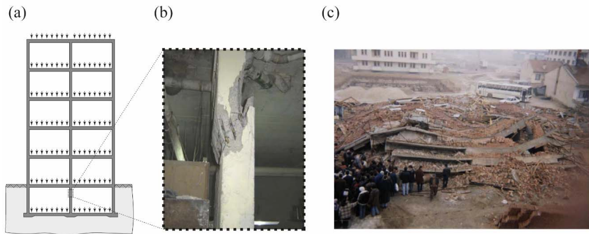
Fig. 2-3 Zumrut apartment building in Turkey: (a) Structural system, (b) heavy damage in the basement columns due to nonlinear creep, and (c) Collapse aftermath (taken from (Kaltakci et al. 2007))
