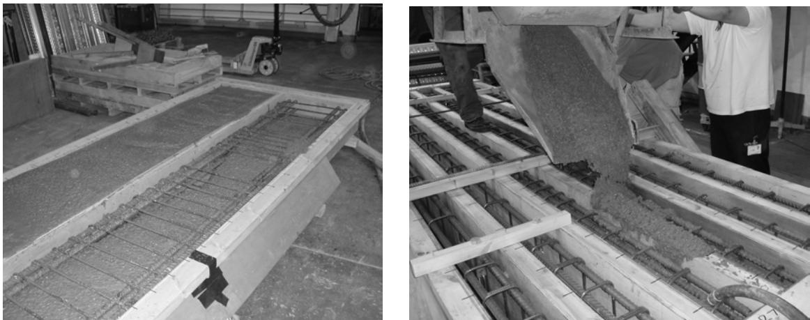
Figure 6.35: Cast of beams B (left) and beams C-D (right)
