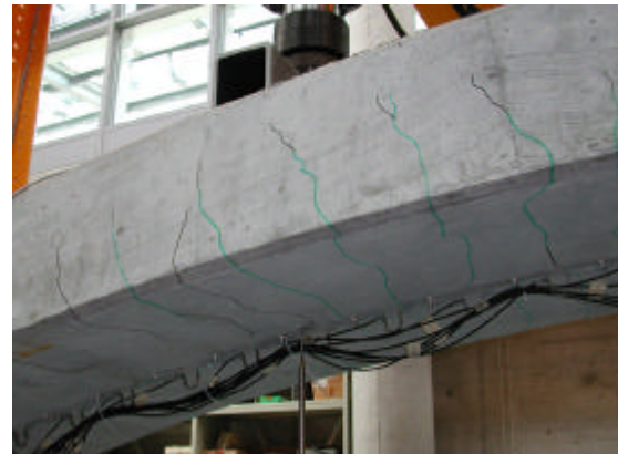
Figure 10. Distribution of cracks in a steel fibres reinforced segment.
